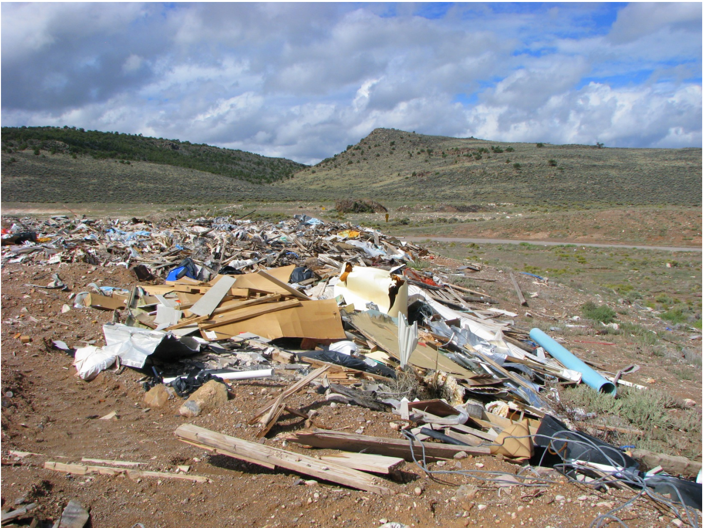
The working face of the construction and demolition waste cell
